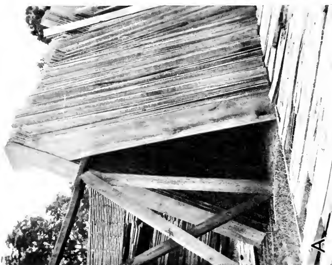
Reasonably good end-racking practice: A, Yard lumber end racked in the form of an inverted V; B, supports for end racking lumber
